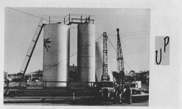
When you don't want a tank, well take it down. The first three petrol tanks at Hawera depot of an oil company to go. This one weighs six tons, stands 36 feet high and holds 9,000 gallons.
